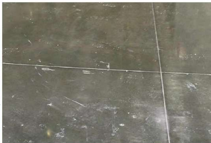
Whitish areas around the construction joints.
