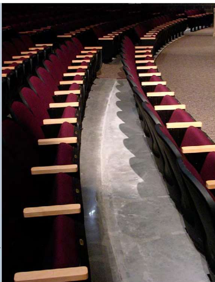
This auditorium at Millstone Township Middle School, N.J., features a combination of carpet and exposed concrete. Joe Smith, Natural Stone Care, Media, Penn., hardened and densified the floor and polished to an 800-grit resin finish.
