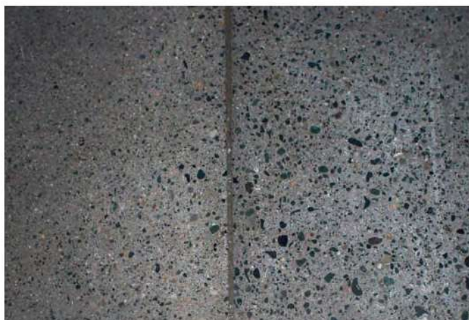
A water-based antique gray stain from Smith Paints turned out to be a perfect match for blending the whitish areas with the concrete.
