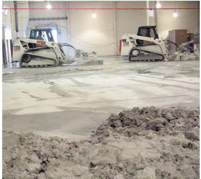
At the Diacon job, modified Bobcat T250s were used to remove Stonhard ATK from a slab in a building once occupied by Tandem Computers Inc.
