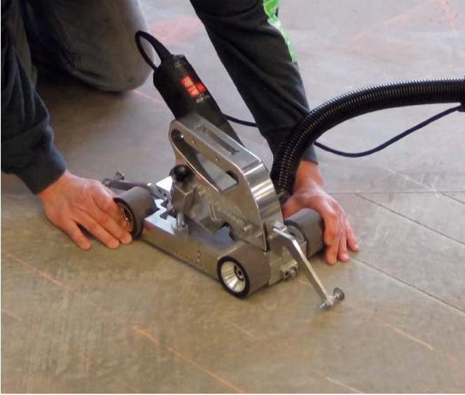
Concrete engraving requires a blade that operates at low horsepower because the goal is to carefully wear away the surface of the concrete rather than make a deep cut.
