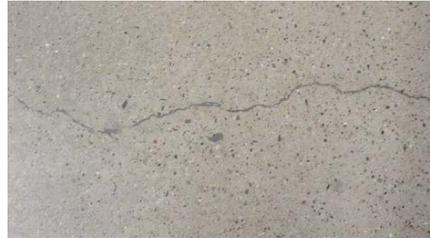
On all the programs Stephenson manages, “filled not chased” is the preferred method of handling cracks.
