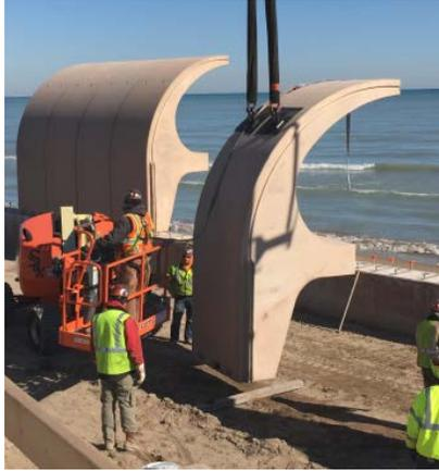
Utility Concrete Products cast 109 five-foot-wide segments, many as tall as 20 feet, to create the desired look. The artistry was completed by coloring the mix with custom-modified Scofield Integral Color SG in Sand Buff and finished with a sandblaster to match the building's limestone.
