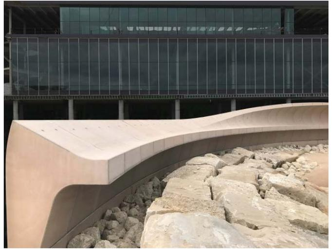
Installation required some creativity, innovation and tight planning. The precast panels were mounted on a cast-in-place kneel wall using both column-base connectors on the land side and splice sleeves on the lake side. This unique system, developed just for this project, allowed the contractor to bolt the panels in place without using an interim bracing system.
