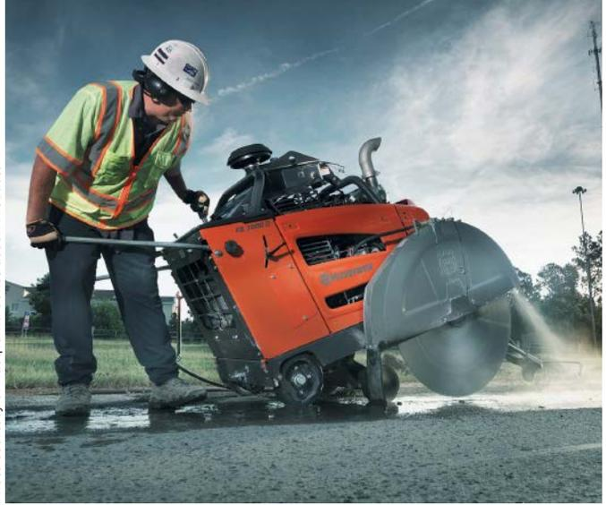
Making large, deep cuts for something such as highway expansion joints requires a blade that can cut many linear feet at high speed.
