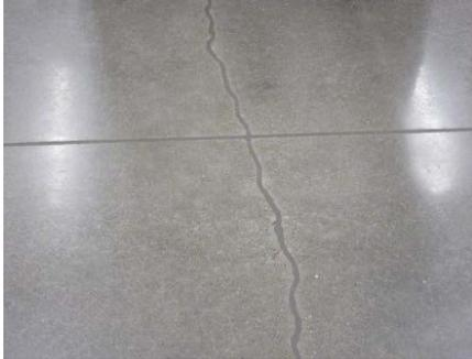
Crack chased and filled
