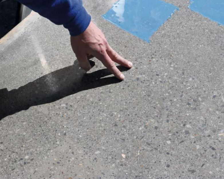
Hi-Tech Systems displayed how stealthy its Spall-TX3 could be. You can barely see where the polyurea concrete repair material was used on this surface as it literally makes the repaired area disappear. This rapid-set, 100 percent solids material is designed to rebuild and repair broken control joints and spalled concrete. On top of that, it's polishable.
