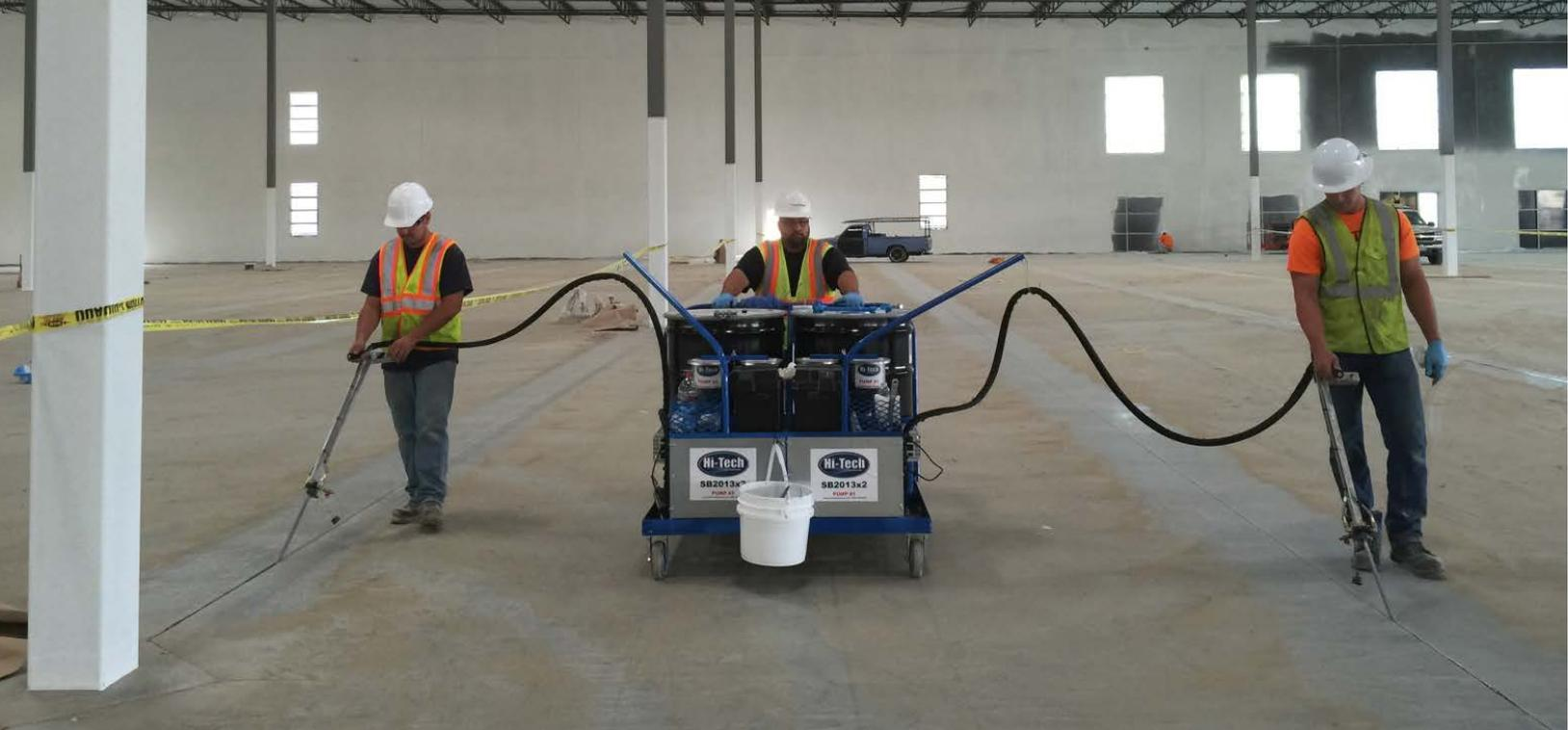
A big job can require big equipment. This large pump, designed especially by Hi-Tech Systems, allows two workers to dispense polyurea at the same time.
