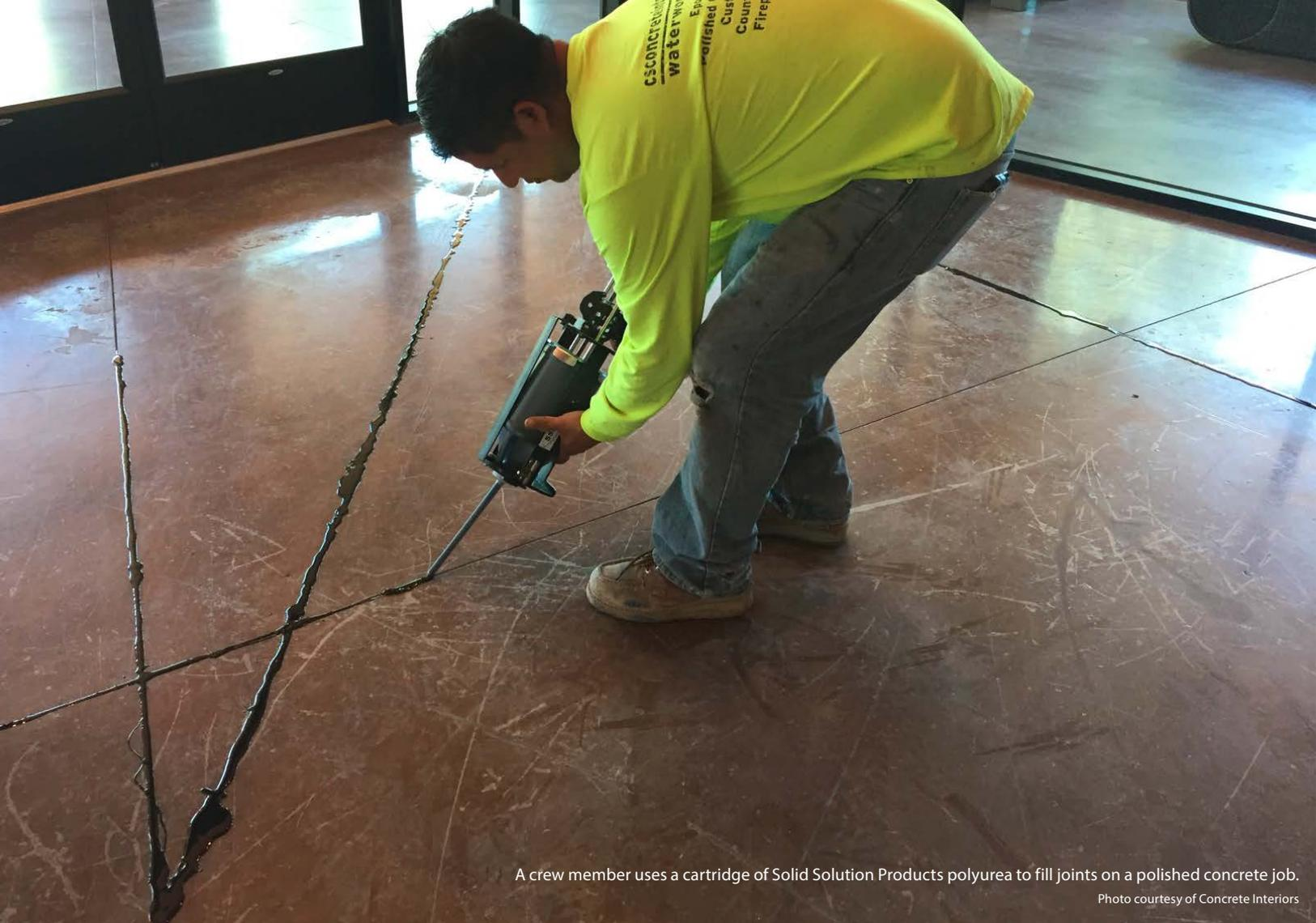
A crew member uses a cartridge of Solid Solution Products polyurea to fill joints on a polished concrete job.
