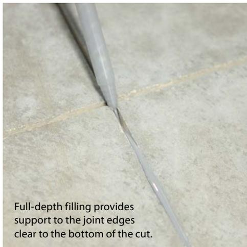
Full-depth filling provides support to the joint edges clear to the bottom of the cut.
