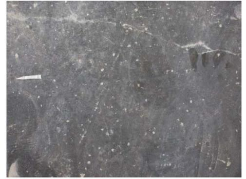
are several hundred thousand screw chips in this high-end floor. All the white dots in this photo are chips in the concrete surface. (See photo above.)
