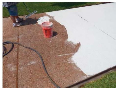
A scratch coat of limestone overlay is applied over pea gravel-exposed aggregate.
