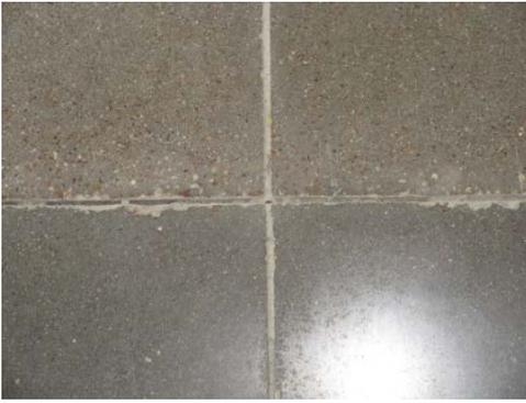
are brought in and out and heavy loads on small tires cross control joints, the edges or shoulders of the joints get broken. This causes spalling as the concrete breaks down which causes more breakage to occur. (See photo above.)
