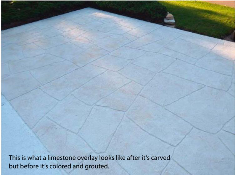
You can use a cement board scoring tool to carve a pattern into a limestone overlay.
