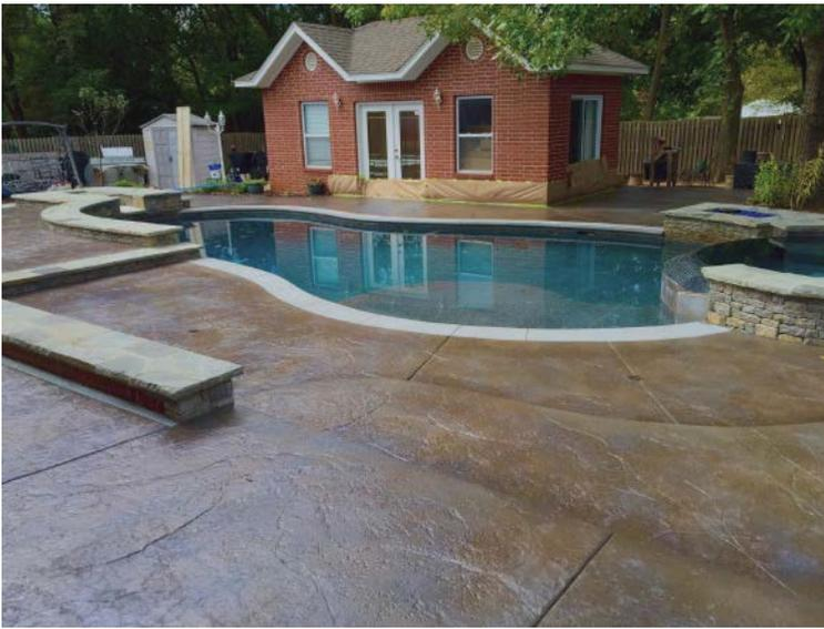
After stamping this pool deck in Broken Arrow, Oklahoma, and staining it with a series of grays and walnuts, Andy Jones applied a proprietary dry pigment mix that gives the surface color-changing qualities. To tie it all together, he then added glow resin around the pool inside control joints and decorative cuts.
