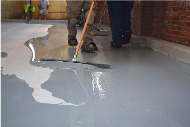
Drytek from Laticrete is Frankel's moisture control barrier of choice because it can be put down in various strengths to control almost any degree of moisture.
