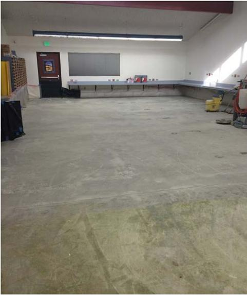
the underlying terrazzo floor, rather than replacing the carpet. Stripping and polishing tests were conducted and the decision was made to restore the original terrazzo floor, saving tens of thousands of tax dollars.
