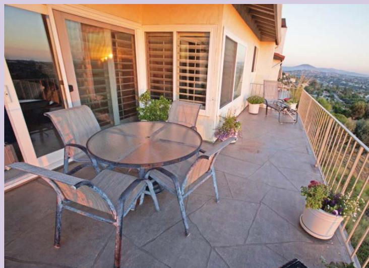
Westcoat's Stone Strips are an applicator's dream when it comes to creating a natural flagstone pattern in decorative concrete overlays. Thanks to the strips' design, no cumbersome tape is involved in the process.
