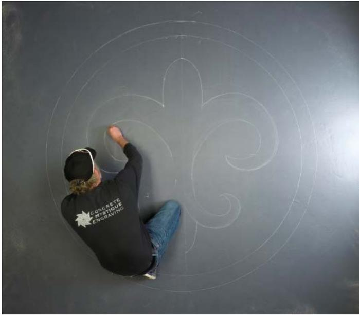
Now you can finish off your curves and separate it into three different parts. At this point, I realized the tips of the center were too plain. I adjusted those tips and finished the image. I now can use the existing shape to my advantage to keep everything centered and consistent.
