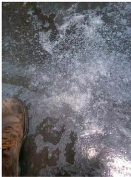
Many contractors are afraid to apply sealer for various reasons. When not applied correctly, problems such as bubbling, flaking and blistering can result.
