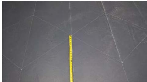
It quickly starts to get easy here. Measure 14 inches in both directions off the initial parallelogram on all your 18-inch lines. Now connect the dots and you'll see the 3-D. Of course, it will be easier to see it once you
