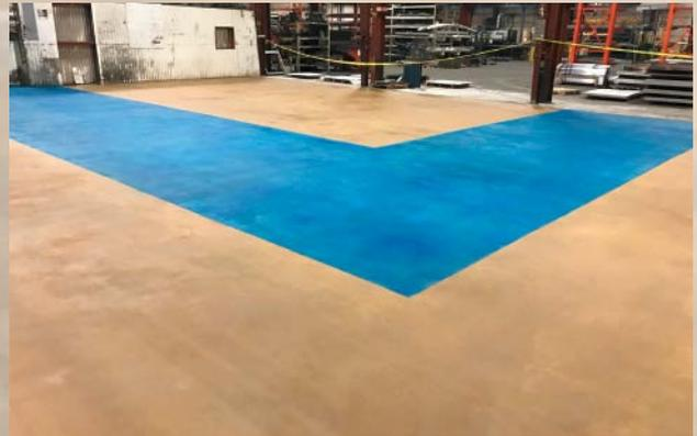
*Endurable Polymer Pavement with sand broadcast and stain*
