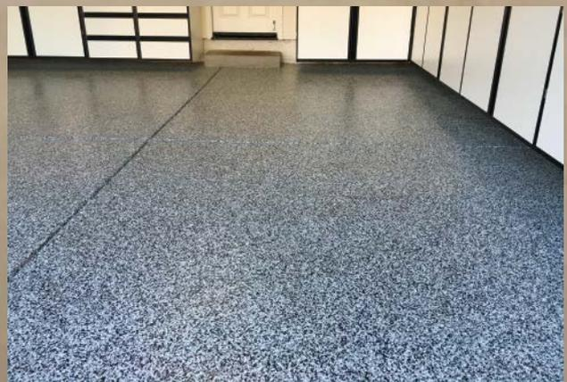
*Endurable Polymer Pavement with Color Chips*
