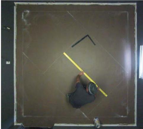
Draw a perpendicular line on the right 18-inch dashes, another 54 inches long. Finally, draw one through the center skipping one section in the middle. When finished you'll have a 3-foot tile, a 54-inch tile, four 36-inch tiles and one 18-inch square. Repeat this layout in every 6-foot box.
