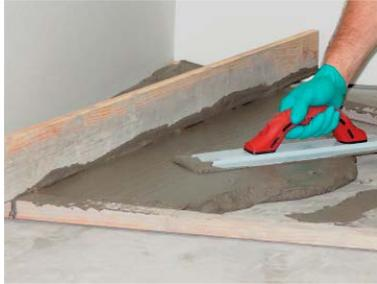
Dur-A-Tex LM is a quick-curing, single-component latex mortar requiring only the addition of water for mixing and use. Dur-A-Tex UM is a three-component urethane mortar supplied as a premeasured kit for simple use on site. Both products are designed for bucket mixing and trowel application and can be applied prior to installing any of Dur-A-Flex's Accelerator, Hybri-Flex, Poly-Crete or Epoxy floor systems.
