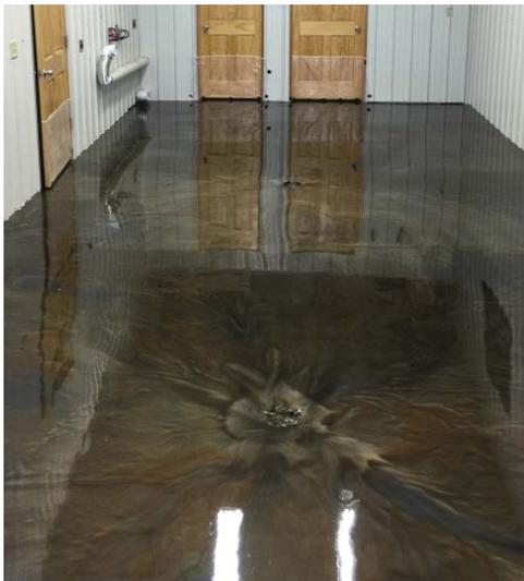
The first coat of PT1 epoxy with the colored metallic additives has cured. Notice how much the Reflector Enhancer has moved from the previous step.
