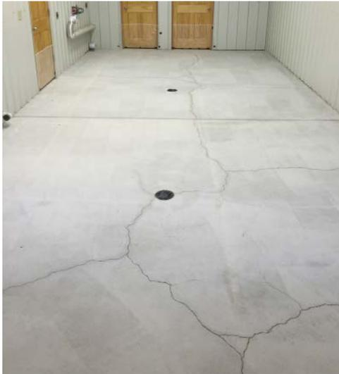
The concrete is ground and the cracks are prepped for a seamless epoxy installation.
