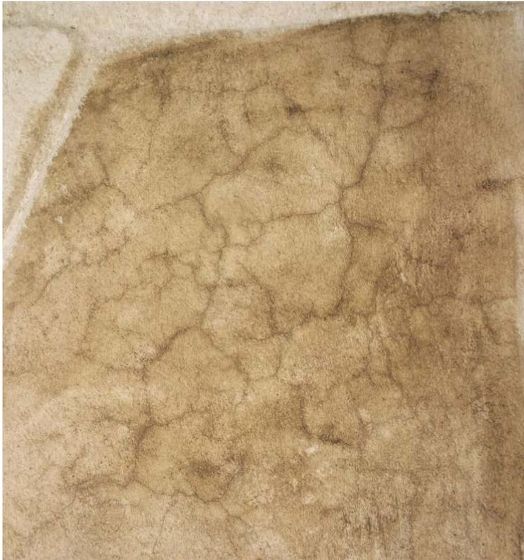
Craze cracks are a network of fine random cracks or fissures on the surface of concrete or mortar that's caused by shrinkage of the surface layer.
