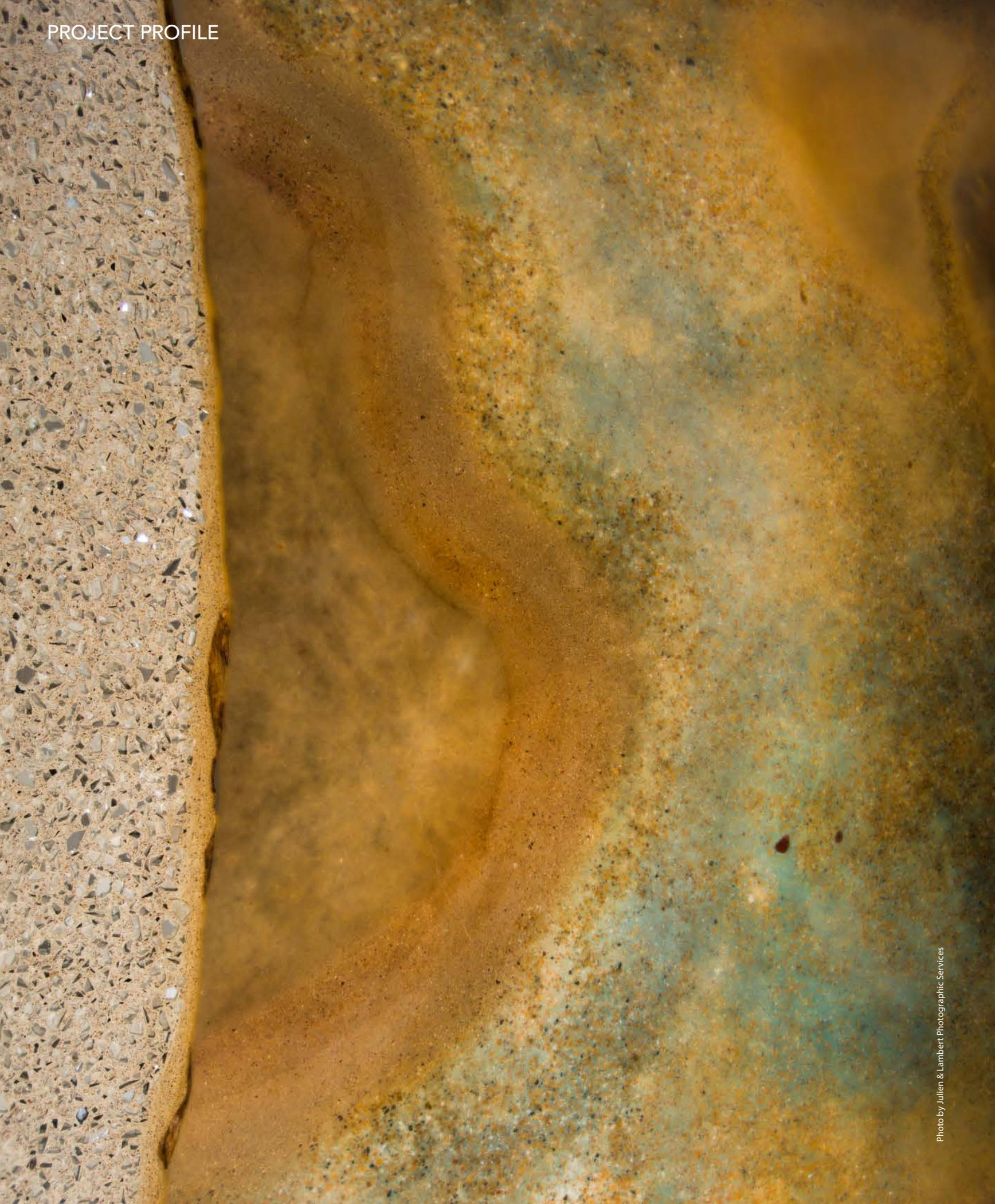
a raised service top with recycled crushed mirror pieces and a chiseled-rock edge.
