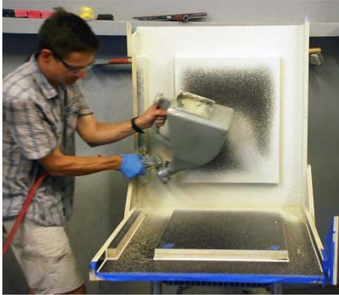
We applied the mist coat using a hopper gun, at a fairly thin thickness of 1/16 inch. Some areas, particularly the corners, were impossible to spray, and we had to apply the mist coat by hand.
