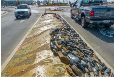
Surrounding the roundabout, 12 islands of various shapes and sizes are fashioned out of a proprietary concrete mix. Each is acid stained in multiple colors and contains starfish, shells, small pebbles and a mix of large flat rock. Acid-stained veins on most of these steep-graded surfaces make them look like vertical concrete, Ralston notes. “To make veins that would not run down in errant patterns everywhere, we had to develop a staining system.”
