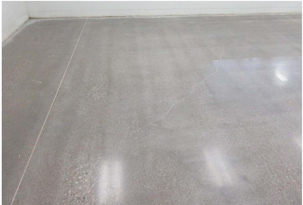
Scratches left from the grinding process are common.
