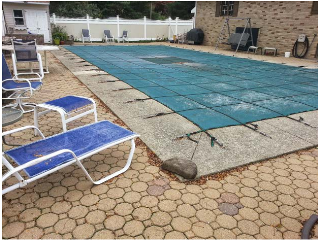
The old pavers had settled, but the concrete pool coping was still in good shape. The Fishers had to maneuver material in the tight space between the pool and the fence.
