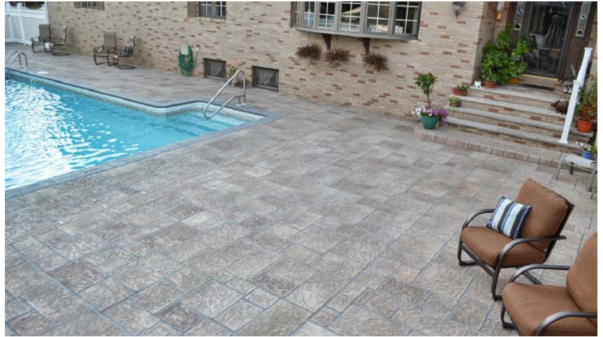
If you look closely, you can see a straight line, which is actually a sawcut, running from the middle of the last step through the pool deck. Also to offset the pattern and draw attention to individual shapes, the Fishers hand-applied various stains to each rectangle.
