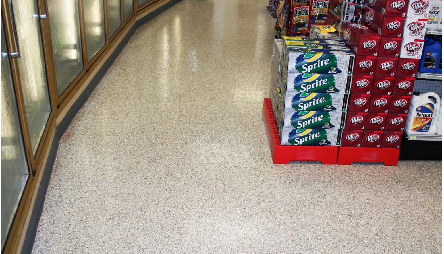
This floor features a double-broadcast quartz system. The client was looking for a decorative floor as well as a surface that was both impact- and slip-resistant.
