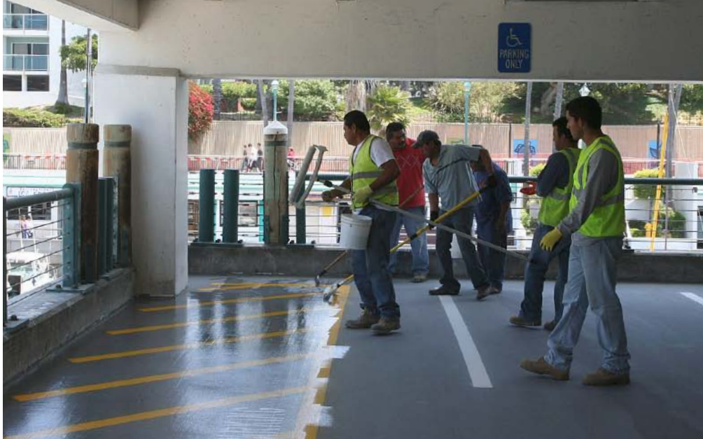
While applying a clear polyaspartic coating over a decorative finish, this crew broadcasts and back-rolls glass-bead aggregate for added slip resistance. The glass-bead aggregate will not take away from the aesthetics.
