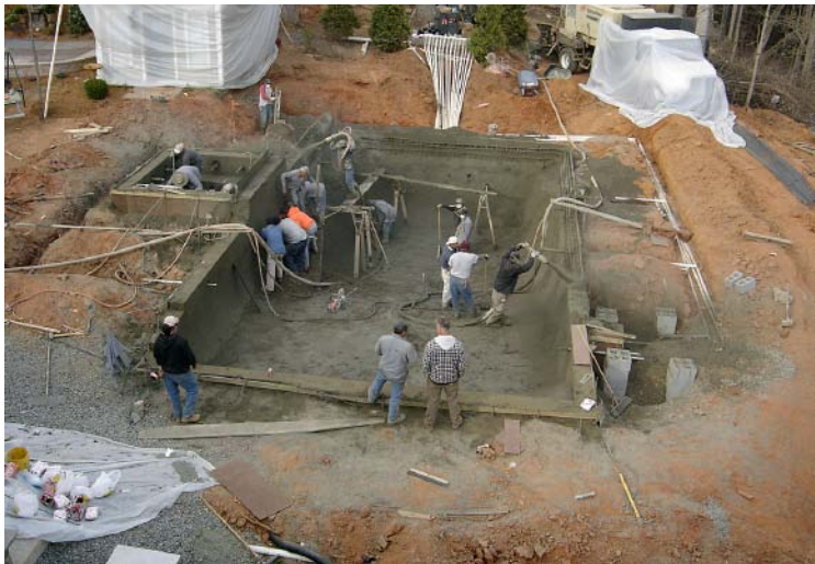
Workers installed 80 yards of shotcrete when constructing the pool.
