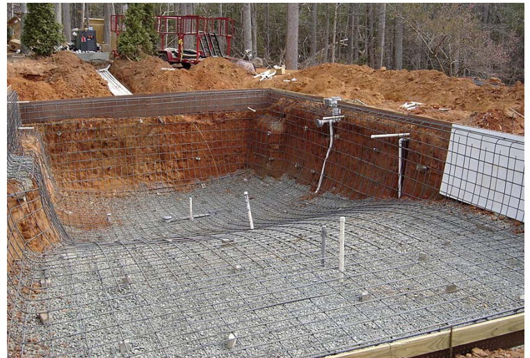
More than 2 1/2 tons of 4-pound rebar were installed 12 inches on center for extra reinforcement in the new concrete pool at the "Hidden Oasis."
