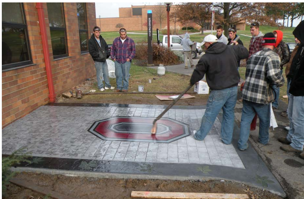
Showing homeowners how to properly apply sealer can save you a lot of headaches down the road.
