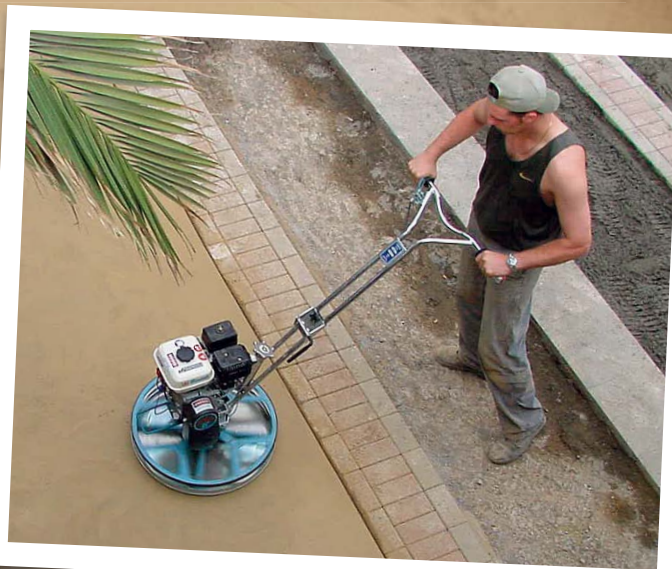
Blast from the past: A young John Anderson operates a power trowel on the North Atlantic island of Madeira. The tree isn't your typical palm — it drops seed pods that permanently stain the concrete.
