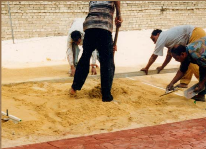
To train workers in Egypt, fine sand was utilized to practice screeding, floating, finishing, and stamping concrete.
