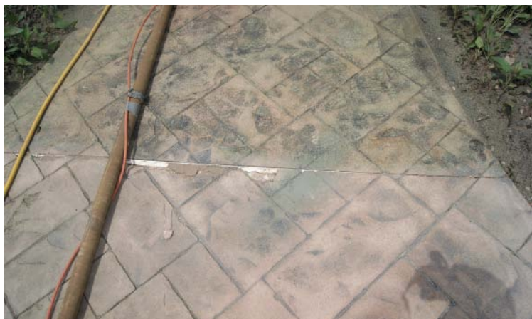
The sandblasted surface on the bottom half is ready to be resealed. As you can see in the top portion, sealer had been overapplied, leaving the surface discolored.
