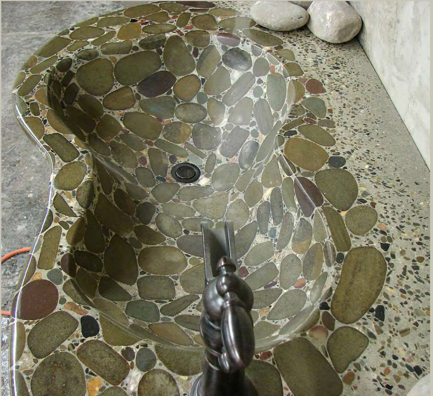
A sink crafted by Mark Celebuski. The cement-rich mix had no problems bonding to inlaid stones.
