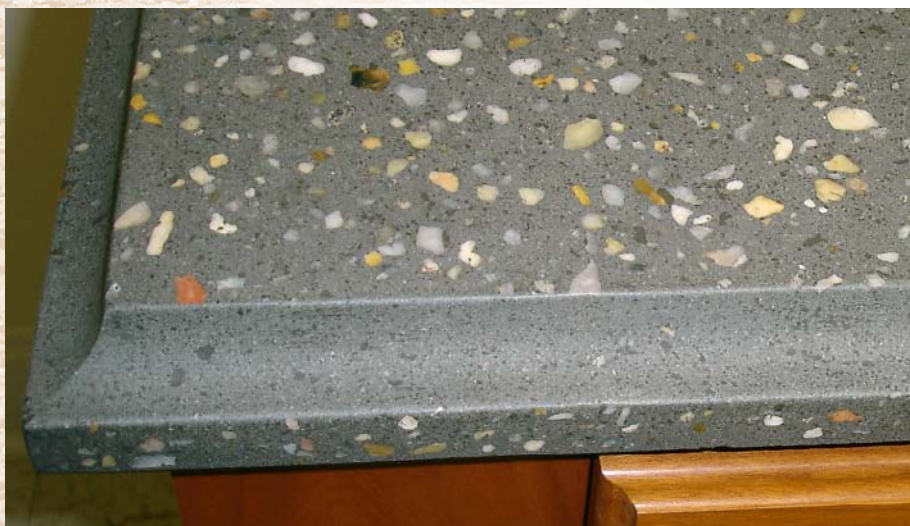
This countertop's flat surfaces were ground and polished to expose the colorful aggregate. The curved edge was formed by casting the concrete against a piece of 3/4-inch round-over molding.
