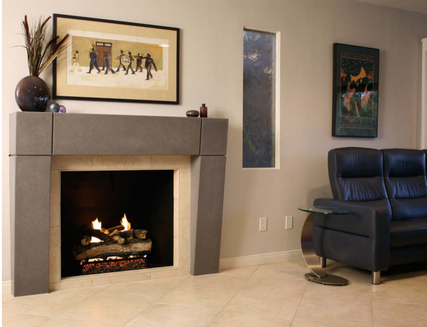
This fireplace from Pourfolio is a single casting with grooves to give it dimension. Because the mantle tilts forward into the room, a French cleat was cast into the piece and attached snugly to the wall. The clients' artwork and the color of their sofa inspired the design.
