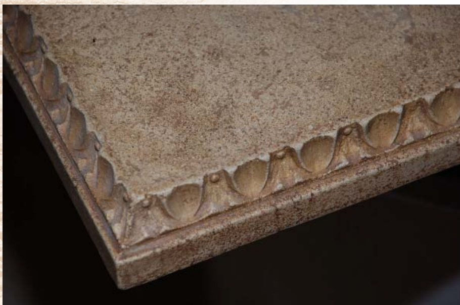
A piece of flexible architectural molding was used to create this traditional egg and dart pattern.
