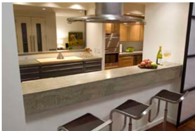
At the Johnston residence: Stone-colored counters, mostly poured in layers to produce stratifications. The kitchen has two bar tops with drop-nose features, and the kitchen counters have integral bamboo cutting boards, trivets and elevation changes.
